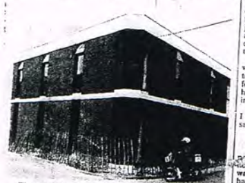
The site on Friday morning — not a workman in sight.
